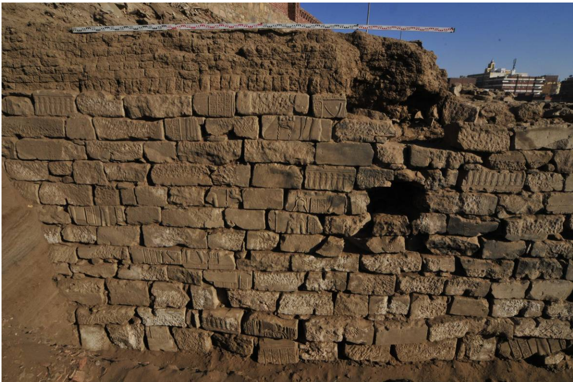
Fig. 9: Area 2: Detail of the southern face of the casing with reused blocks.
