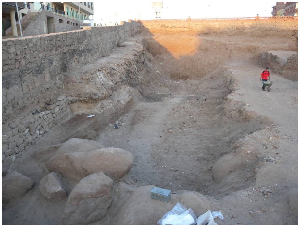
Fig. 3: Overview of the excavated foundation pit.
